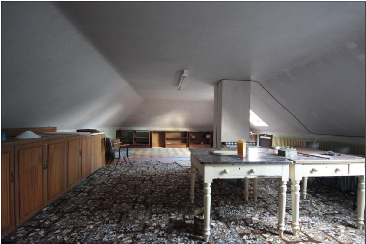
Plate 14: Attic level of the single-storey front block of the former convent.
