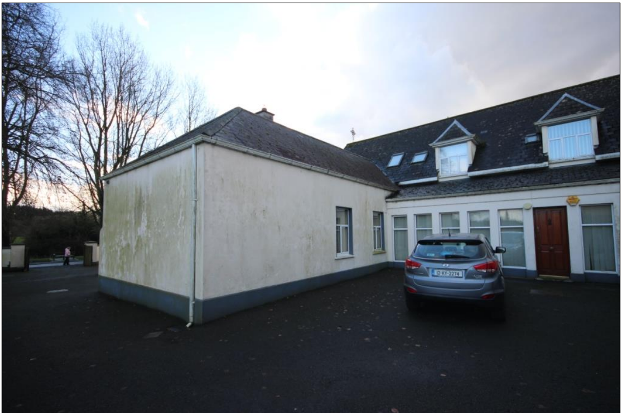
Plate 4: View of the rear elevation of the original single-storey element of the former convent. The dormer extension to the rear (on the left of the photograph) is a later twentieth-century addition.
